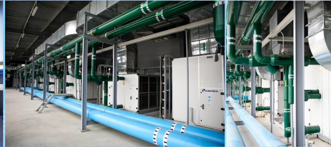
ACTUAL CONSTRUCTION OF HVAC SYSTEM
