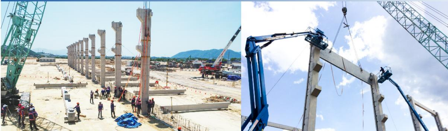
ERECTION OF PRECAST CONCRETE COLUMNS, WALL PANELS
