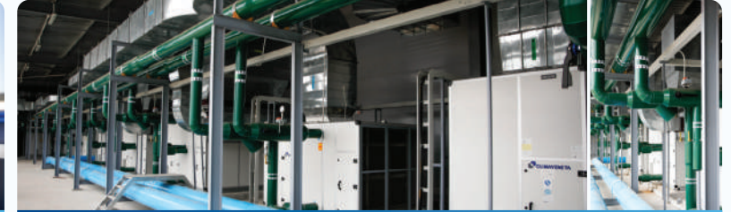
Actual Construction of HVAC System
