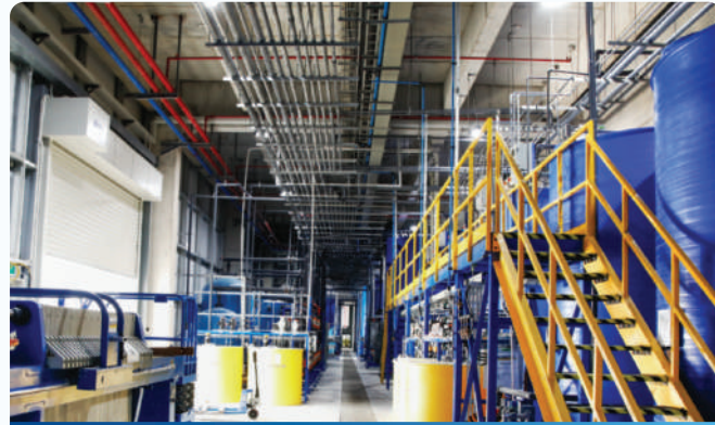
Actual Construction of Wastewater Treatment System
