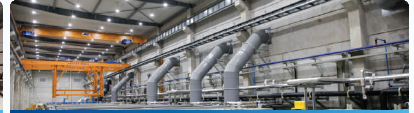
Actual Construction of Anodizing Technology System
